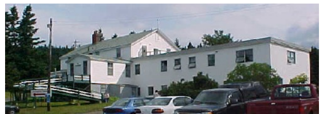
Julia Ann Walsh Heritage Centre provides a good opportunity to strengthen this commercial node
