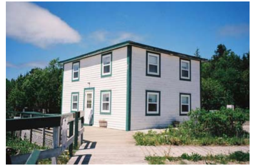
Jenniex House Municipal Heritage Building
